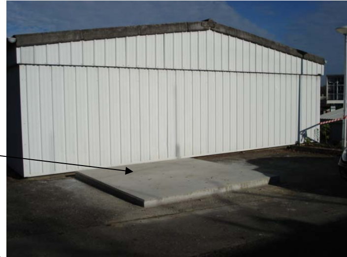
Concrete platform for dewar
