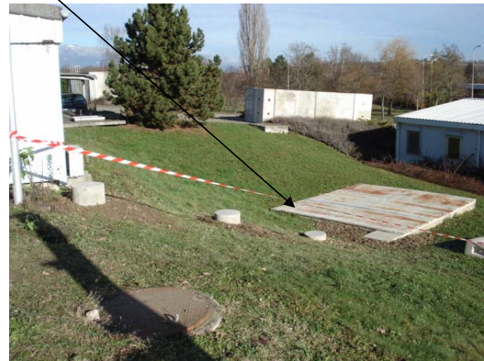
Concrete support posts for transfer line
