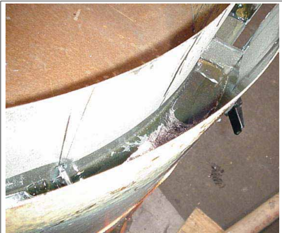
Casting the fillers
