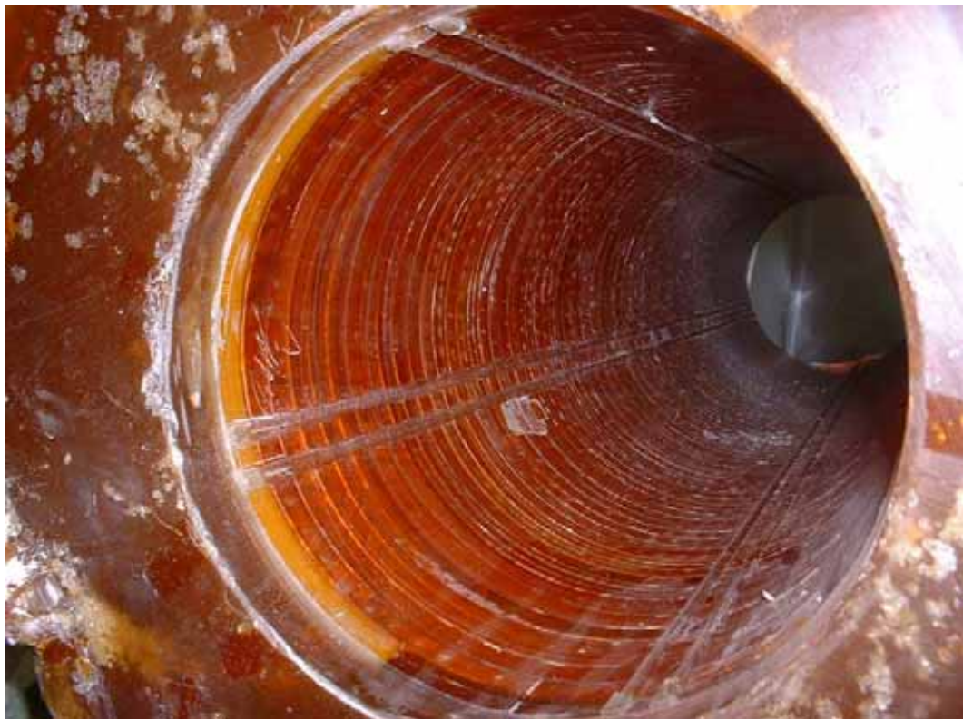
Segment #1 Bore – Will be fitted to CVIP's Bore tube
