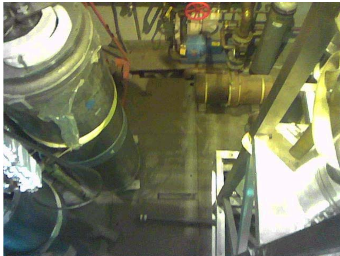
View of the test area floor. The dewars at left and HCX components at right need to be removed
