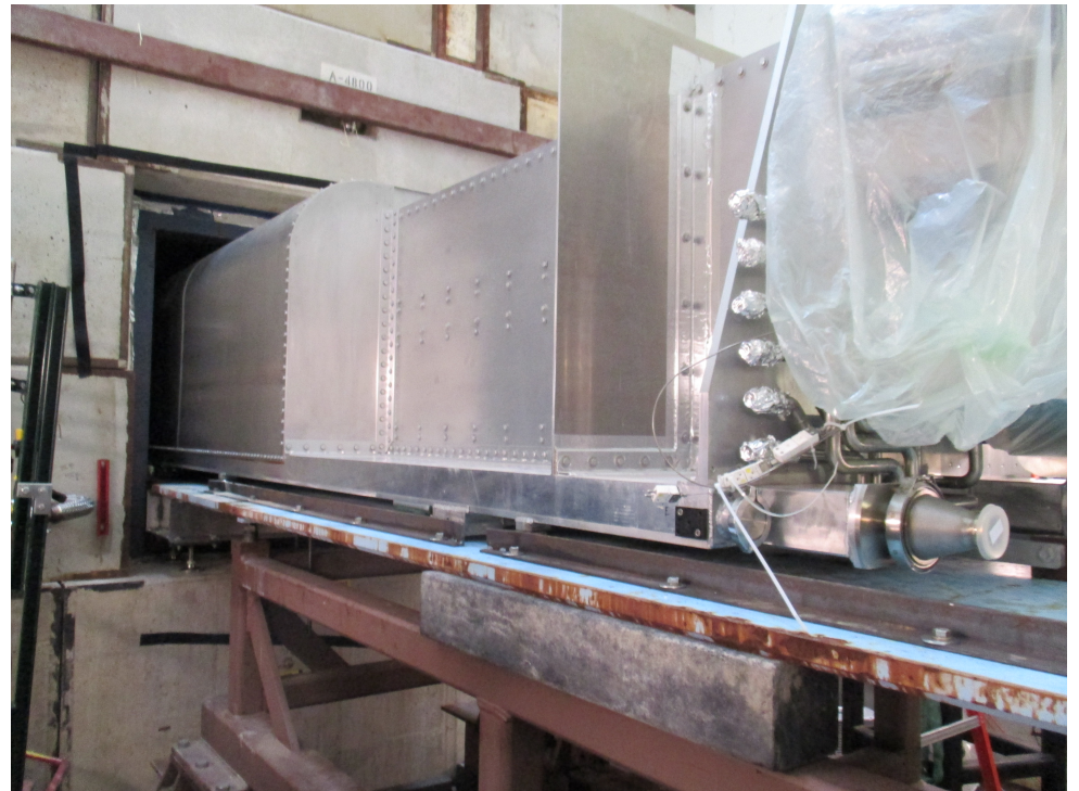
BNB-3 Installation into Target Cave
