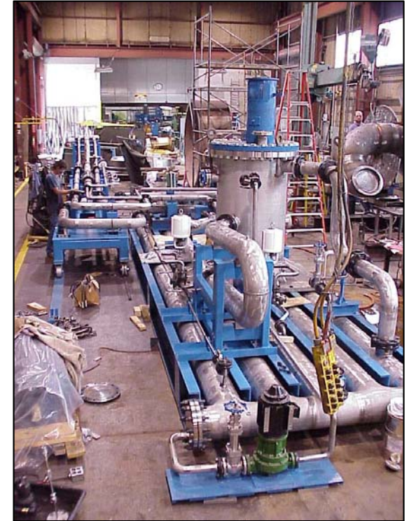
Target Test Facility Hg flow loop during construction
